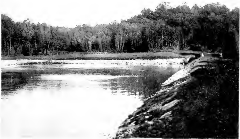
THE SETTLING BASIN.
